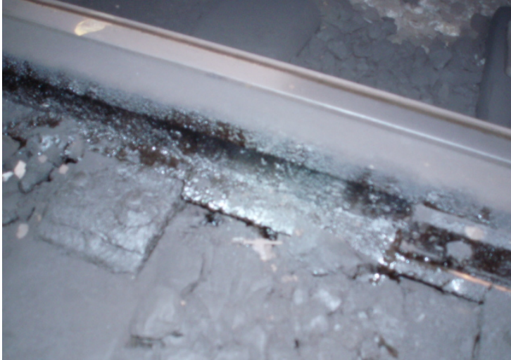
13. View of curve grease on train railway.
